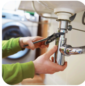
B&L Staley Plumbing Billy Staley 828-442-9946
