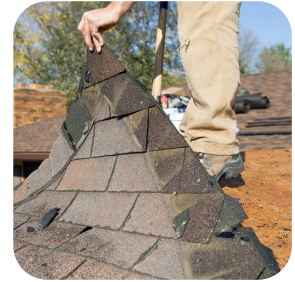
J&J Repair (Roofing and More) Greg Martinson 828-989-9136
